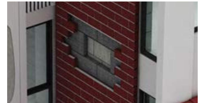
Cavity Wall Insulation Suggested Product: STYRO Graypor 180
