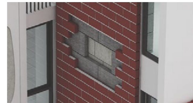
Cavity Wall Insulation Suggested Product: STYRO Graypor 180
